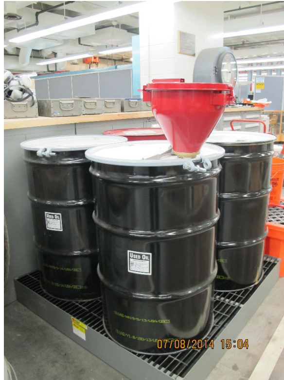
Figure 17: Oil Disposal Drums, showing fire-proof funnel in the foreground
