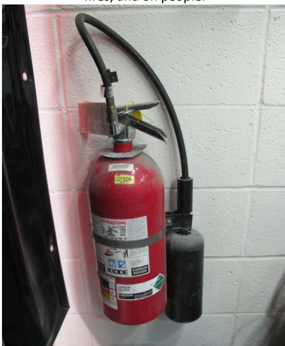
Figure 13: BC Fire Extinguisher with the typical large cone spray nozzle
